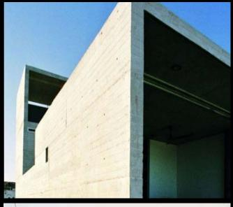
High temperatures, saltpeter, and unskilled labor force were the conditions to decide that this house should be built in concrete. This became the project's starting point, and the tectonic and morphological possibilities of the material followed on the formal definition of the proposal.
