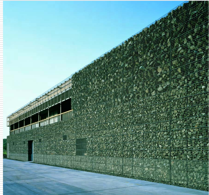
Detail of the facade: a structure in steel wire forms large cages filled by irregular stones.
